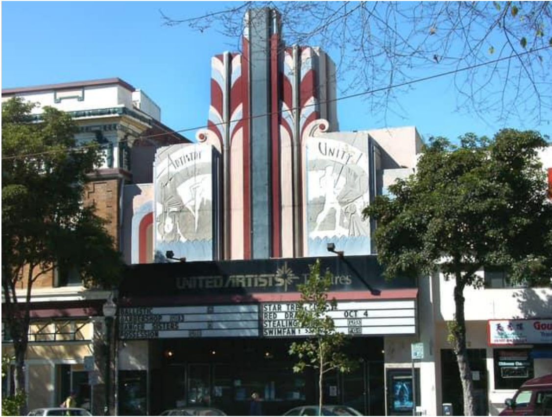
Front marquee and facade featuring the WPA-style Artistry and Unity motif, 2002.
